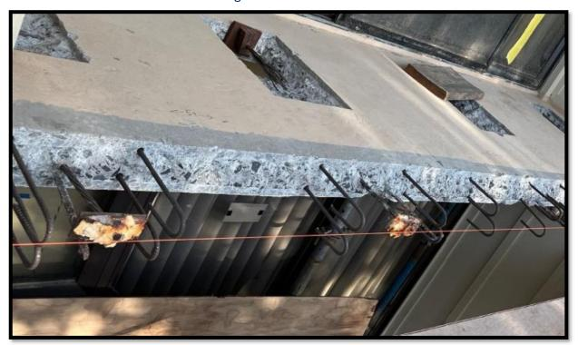
• Cable end caps patched and column repairs at G4 lanai
