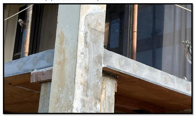
• Temporary lock-offs for cable end repair
